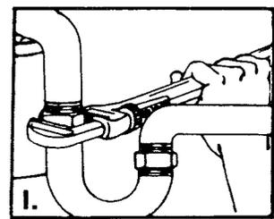
*If it fits* - simply tighten the slip nut on the trap with a pipe wrench to make your connection to the discharge tube complete.
