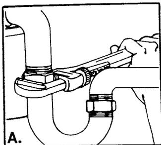
A. Use a pipe wrench to disconnect the drain line where it attaches to the disposer discharge tube.
