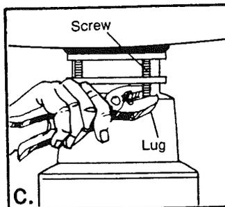
C. If your old disposer has a different mounting than your new one, use a pliers or adjustable wrench to remove the nuts on the mounting ring. Then remove old disposer. (Some disposers have to be removed by taking off a clamp or by twisting the disposer to remove it from its mounting. Easy to figure out.)
