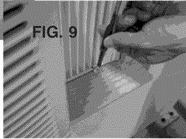
**5** Drive 1/2" (13 mm) locking screws through frame holes into window sash (FIG. 10/11).
