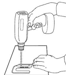
To mount anti-tip bracket to concrete or ceramic floor, use a ⅜" (4.8 mm) masonry drill bit to drill 2 holes at the positions marked on the bracket template. Remove template from floor.
