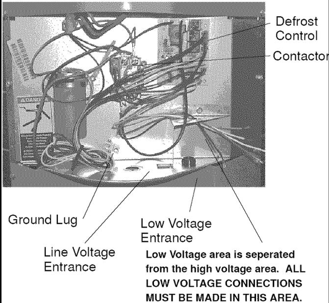
**Figure 10** A/C Condenser Typical Low Voltage Connections
