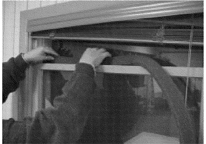
2. Holding the sash down behind the back of the Top Rail (as shown) attach the safety lock. (You may wish to pre-drill a pilot hole using a 1/8" diameter drill.)
