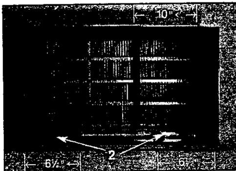
2. Attach (2) Tapered Spacer Blocks to the inside of the wall sleeve as shown in the illustration. DO NOT CUT THESE BLOCKS.
