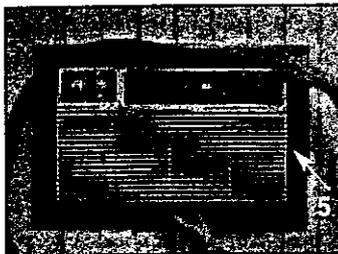
5. Install the 1" x 1½" x 84" long stuffer seal between the wall sleeve and the unit. A flat bladed screwdriver or putty knife is recommended.
