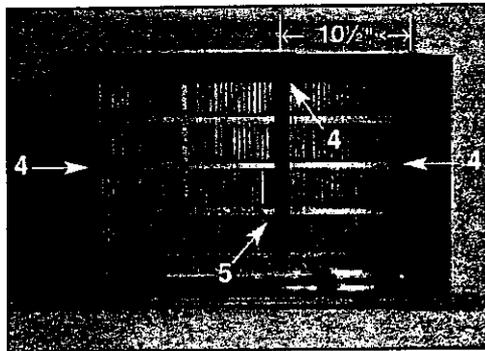
4. Attach (1) 1 1/2" x 1 1/2" x 26 1/2" long seals and the (2) 1 1/2" x 1 1/2" x 14" long seals as shown in the illustration.
