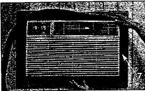
7. Install the 1" x 1 1/2" x 84" long stuffer seal between the wall sleeve and the unit. A flat bladed screwdriver or putty knife is recommended.
