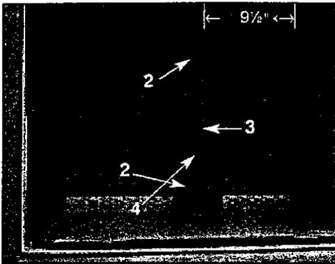
2. Attach the (2) 4½" x 3½" x 1½" foam blocks to the inside of the wall sleeve as shown in the illustration.
