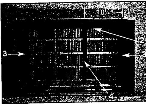
2. Attach (1) 1 1/2" x 3/8" x 26 1/2" long seal as shown in the illustration.
