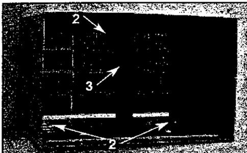
2. Attach the (2) 4½" x 3½" x 1½" foam blocks to the inside top and bottom of the wall sleeve with the slots 10" from the right side wall of the sleeve. Attach (2) Tapered Spacer Blocks behind rib on inside bottom of the wall sleeve as shown. Taper towards the rear of the sleeve.
