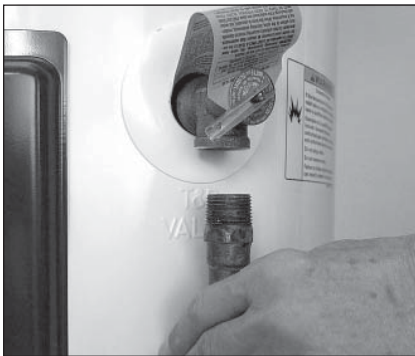
Figure 11 - Removing the T&P Relief Valve discharge pipe.
