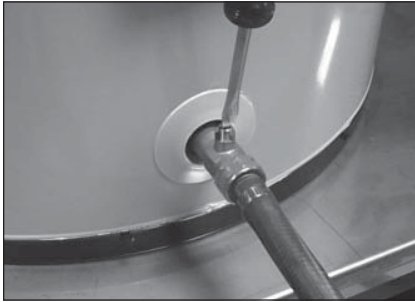
Figure 10 - Draining the old water heater.
