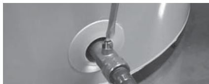
Figure 31 - Drain Valve
