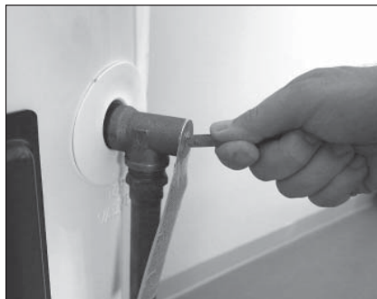
Figure 43 - T&P Relief Valve
