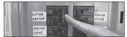
Figure 36 - Circuit Breaker
