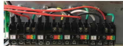
Indoor Unit Power and Comm Wiring
