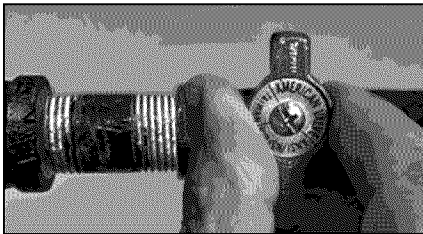
Figure 50 - Gas valve in “off” position.
